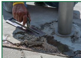
**2** APPLY THE MIXTURE USING A FLOAT OR TROWEL
